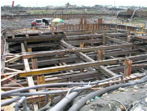
Fig. 9 Picture of test site
