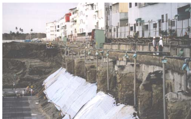
Fig. 6 Deep wells installed near perimeter wall
