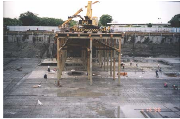
Fig. 14 Completion of stage 2 excavation (south side, main entrance)
