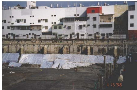
Fig. 15 Completion of stage 2 excavation (east side, adjacent buildings in the background)
