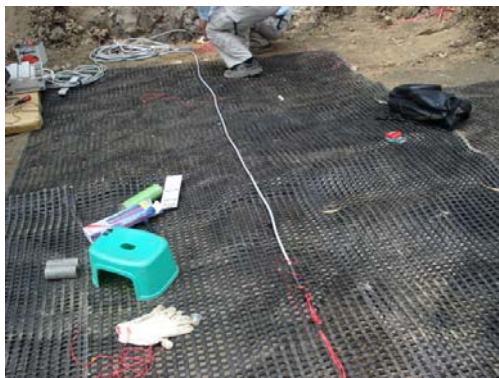
(c) Installation of reinforcement placed with strain gages
