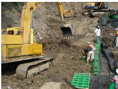
(a) Building embankment facing
