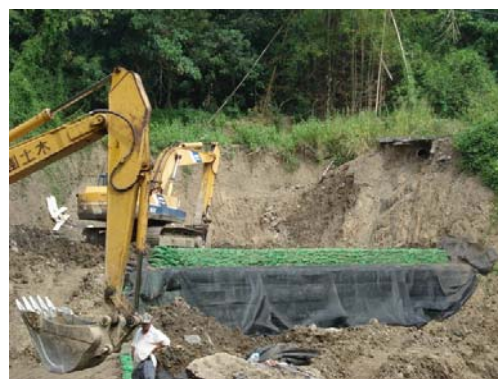
(b) Backfilling
