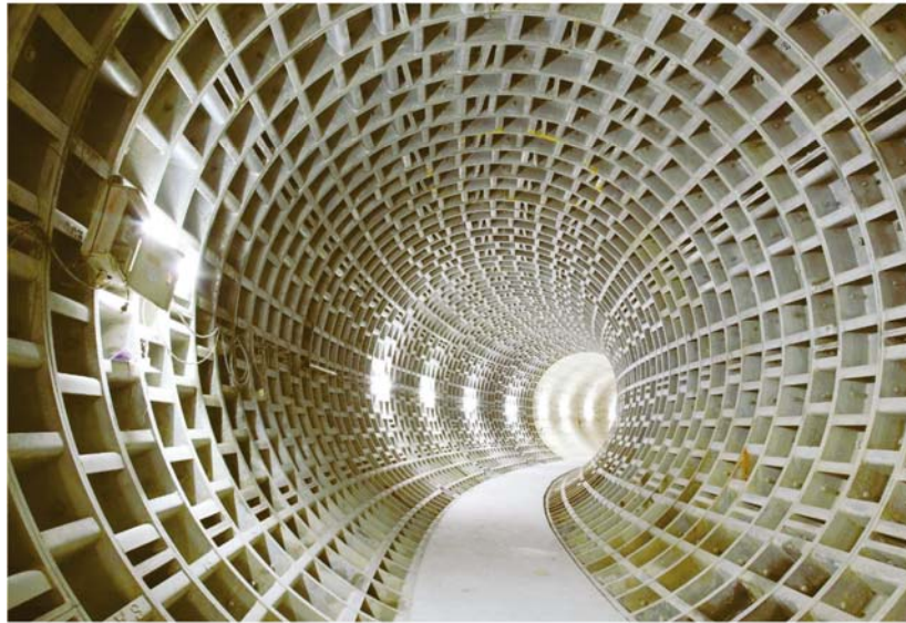
Fig. 13 Steel segments in the sharp-curved section of the tunnel
