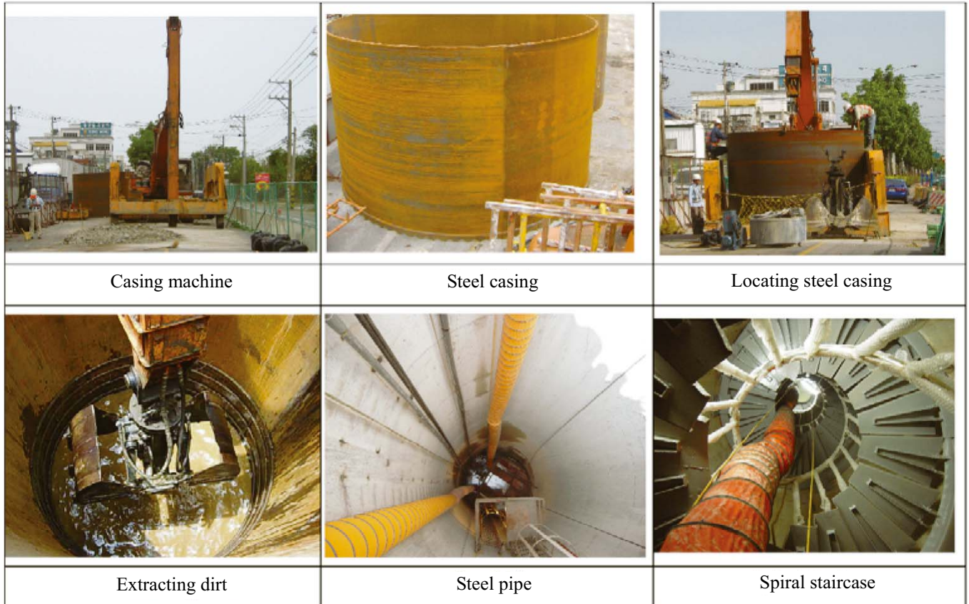
Fig. 11 Steel pipe construction of the emergency exit
