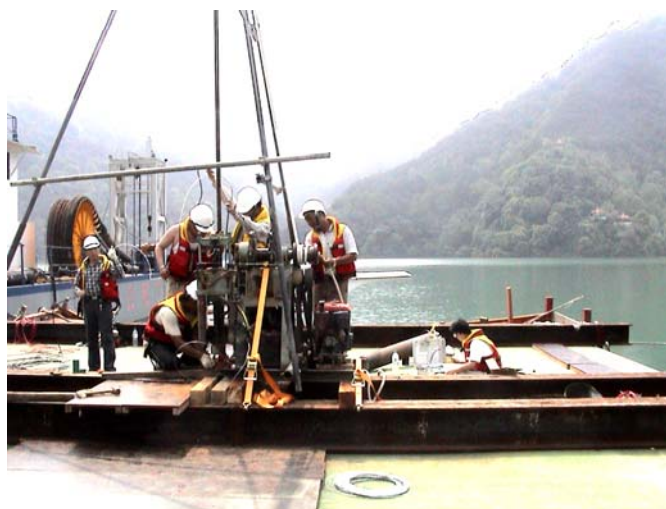
Fig. 8 Operation of TDR/DMT from a barge
