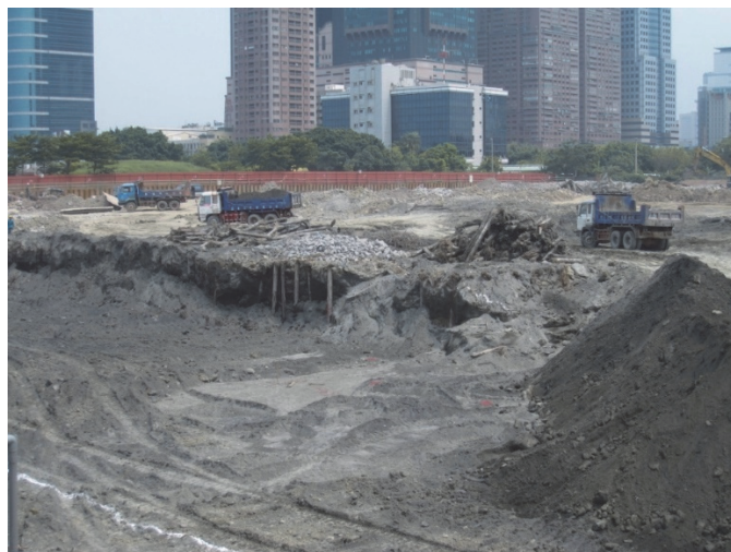
Fig. 6 Timber piles underneath old footings in loose sand
