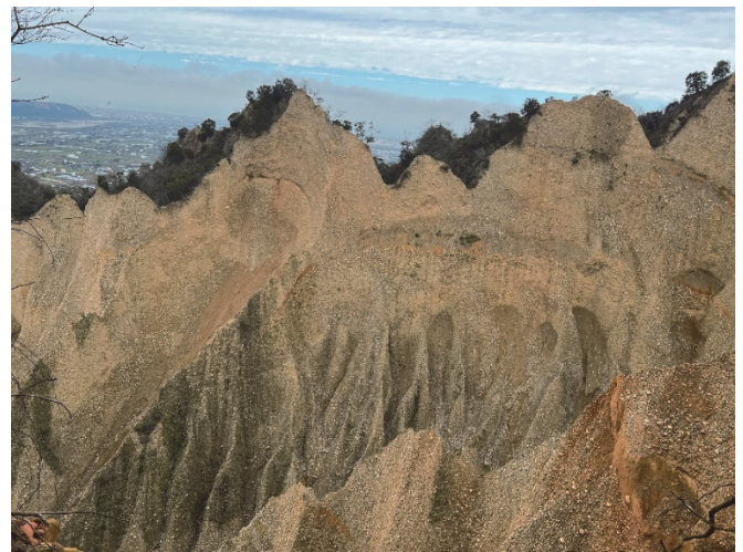
Fig. 1 The Toukoshan Formation—A typical of gravelly soils in Taiwan
