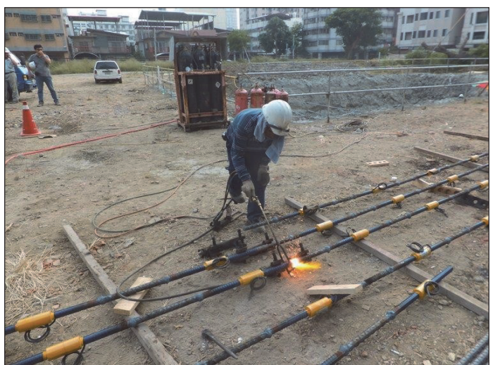
Fig. 9 Rebar strain gages of the test pile
