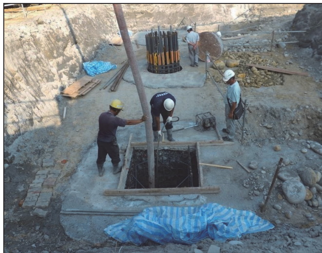
Fig. 8 Construction of the reaction pier
