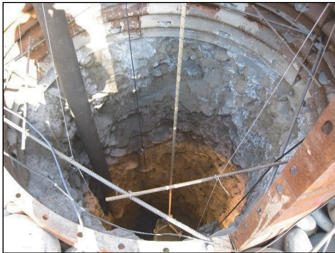
Fig. 6 Construction of the hand-dug caisson (1)
