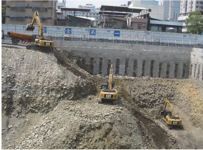
Fig. 3 Typical deep excavation in Taichung
