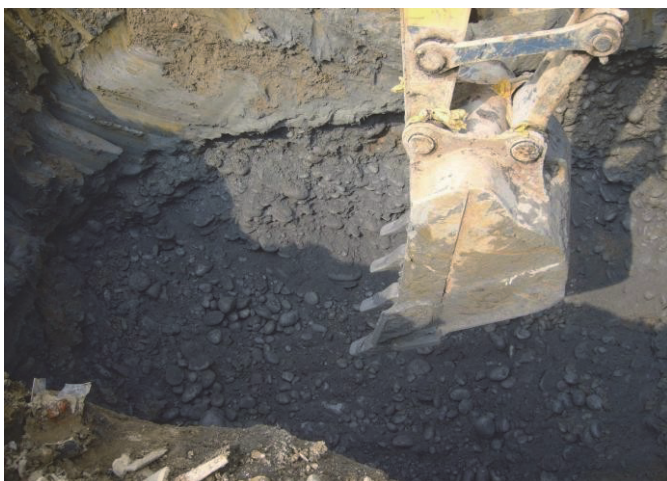
Fig. 1 Test pit excavation
