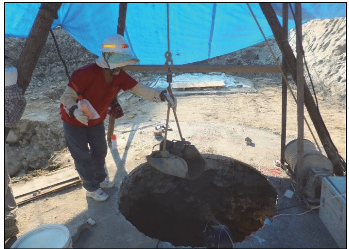
Fig. 7 Construction of the hand-dug caisson (2)
