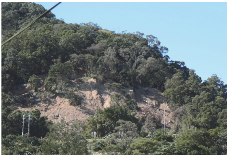
Fig. 3 The condition of the slope after the collapse (Land Engineering Consultants Co., Ltd. 2008)
