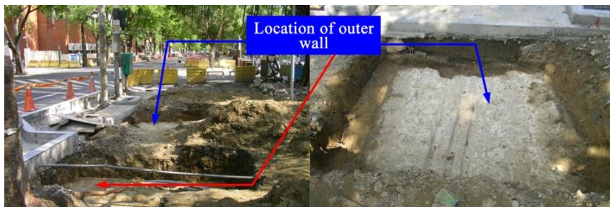
Fig. 12 Outer wall foundation discovered based on Line 4 and 5 GPR images
