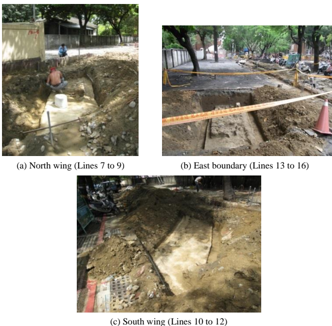
Fig. 14 Underground outer wall foundations by in-situ excavations
