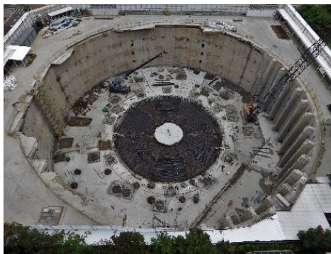
Fig. 8 Photo of the new tube-like retaining wall structure
